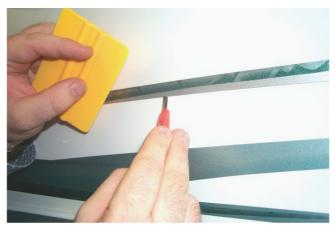
8. If any small bubbles appear during installation, they can be removed by pricking the base of the bubble with the knife blade and squeezing the trapped air out with the tip of your finger.
