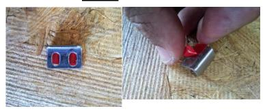
Use a 1/16" drill bit to drill pilot holes using the template as a guide. If the template was properly aligned, the pilot holes should exit slightly above and to the left and right of the push catch latch.
